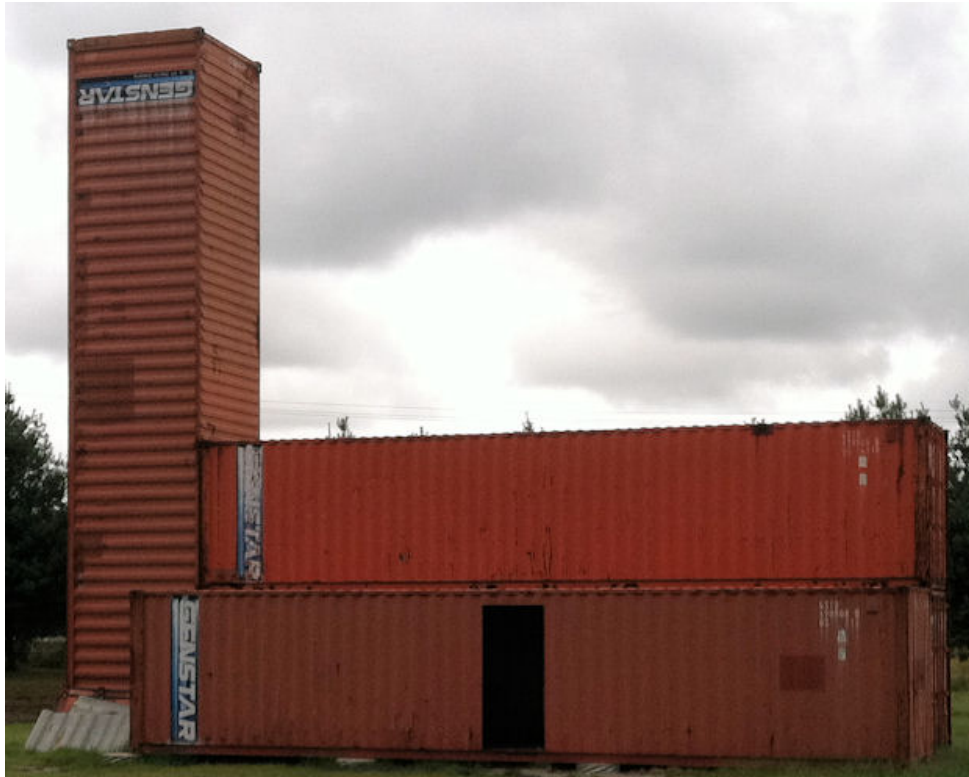
Figure 7 – Sparta Fire Department Training/Burn Building Front Side
