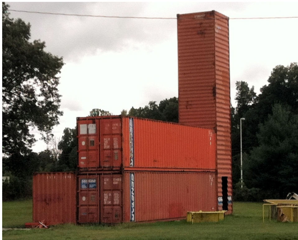
Figure 8 – Sparta Fire Department Training/Burn Building Rear Side
