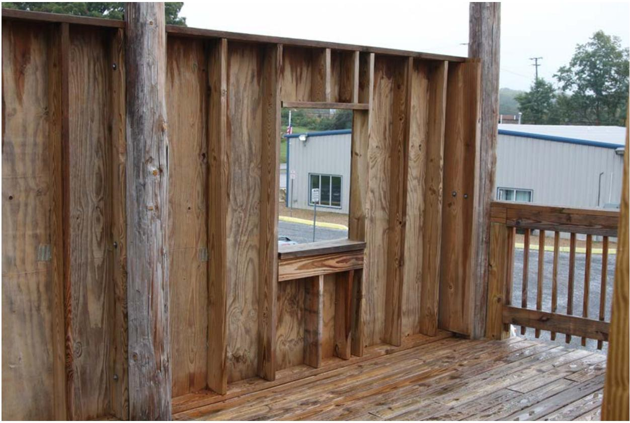
The second floor of wooden drill tower showing the window opening for ladder placement evolutions and the floored work area of adequate size for firefighters to stand and work.
