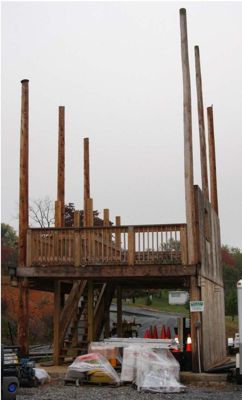
Three story drill tower under construction. Built-in stairs allow hose advancement drills and easy access to the upper floors.
