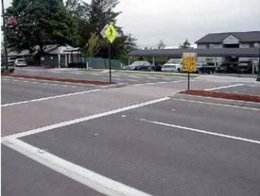
Figure 6. Example of a Textured Pavement Crosswalk. From www.pedbikeimages.org / Dan Burden. Reprinted with permission.
