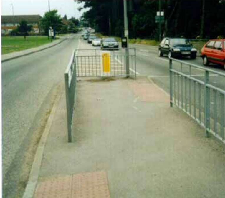
Figure 12-8. Photo. Staggered crosswalk with fencing.
