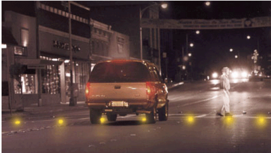
Figure 16. In-Roadway Warning Lights at a Mid-block Crosswalk. From www.pedbikeimages.org / ITE Pedestrian Bicycle Council. Reprinted with permission.
