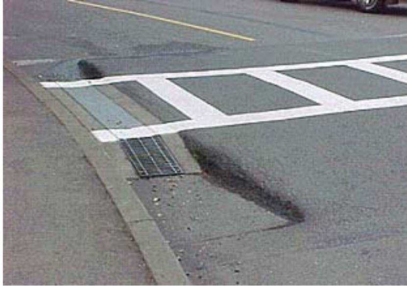
Figure 5. Raised Mid-block Crossing. From http://pedbikeimages.org/ Portland Office of Transportation. Reprinted with permission.
