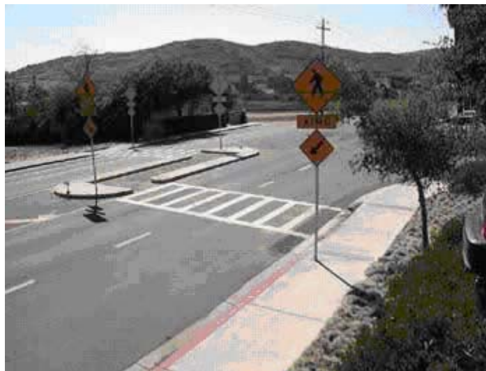
Figure 11. Example of a Split Pedestrian Crossover. From www.pedbikeimages.org/ Dan Burden. Reprinted with permission.
