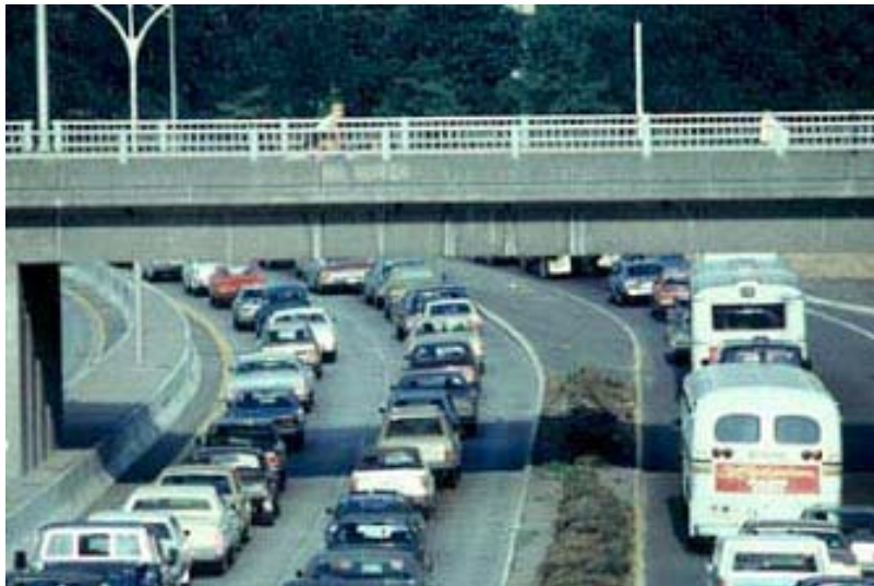
Figure 18. Grade-Separated Crossing (Bridge) Over a Major Highway. From www.pedbikeimages.org/ Dan Burden. Reprinted with permission.
