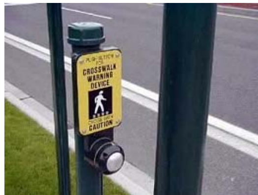
Figure 15. Pedestrian Pushbutton for Flashing Beacon Operation. From www.pedbikeimages.org/ Dan Burden. Reprinted with permission.
