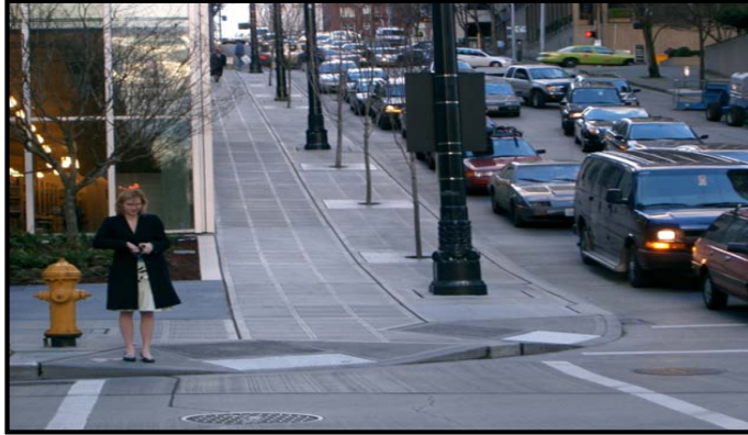
Running slope - can follow adjacent roadway grade
