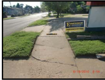
Cracking
