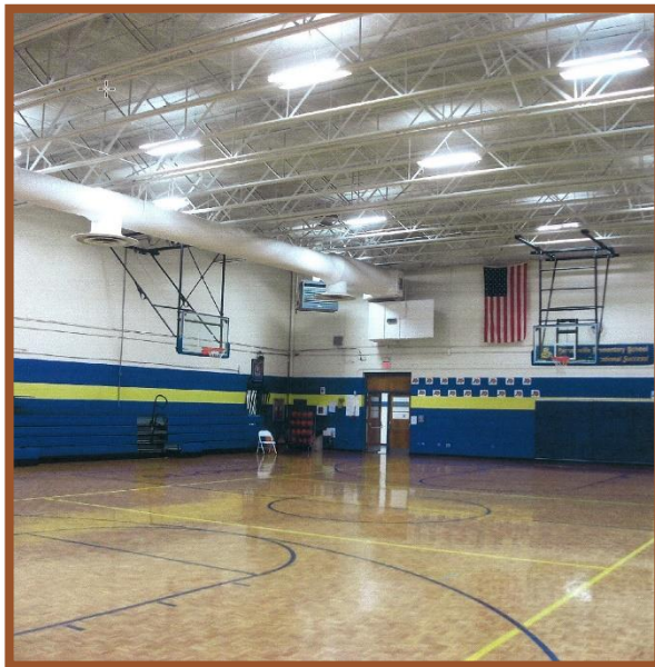
Parrottsville Elementary School — Gymnasium
