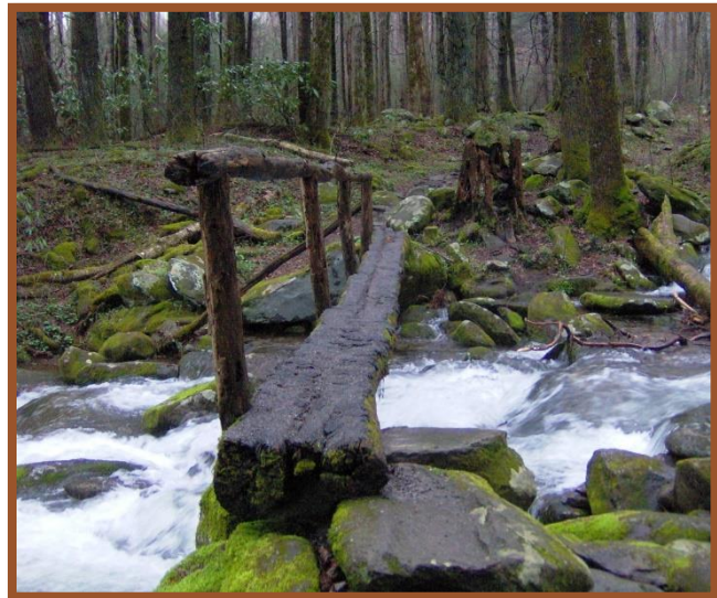
Trail Crossing Cosby Creek in Cocke County
