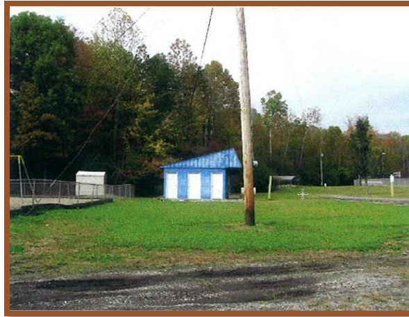
Northwest Elementary School — Restroom at Ballfields
