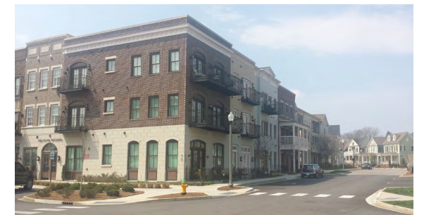
First floor of building reads as the base
