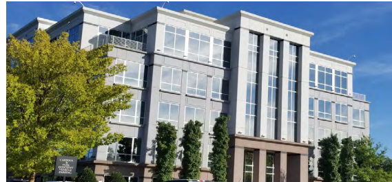
Elements used to reinforce the verticality
