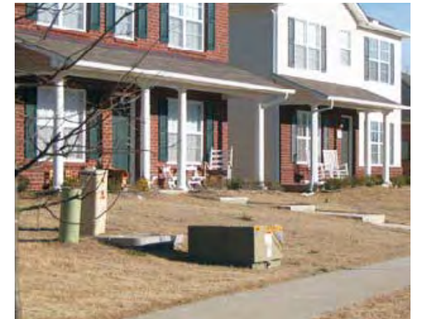
Utility boxes and pads should be consolidated at locations that can be screened (every 4-6 lots). This picture depicts inadequate screening
