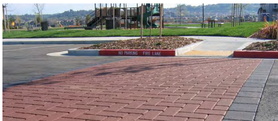
Typical paving Pattern for Pedestrian Crosswalk
