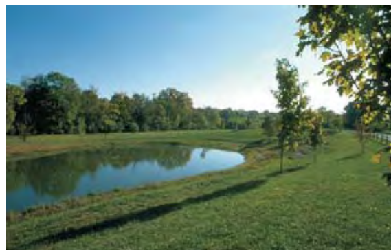
Retention Pond in Open Space
