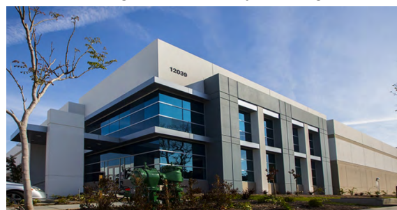
Mix of tilt-up concrete and architectural metal panels on industrial building
