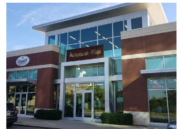
The building base is expressed with a different masonry material. The base at the storefront is expressed with an 8” raised bottom mullion.
