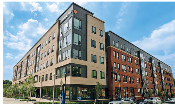
Use of variety of brick colors and cementitious panels on residential / commercial building
