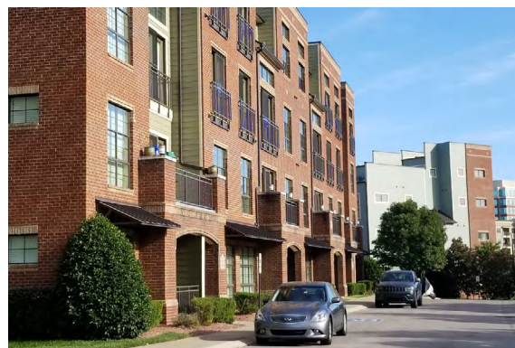
Mix of Brick and cementitious siding on multi-family building
