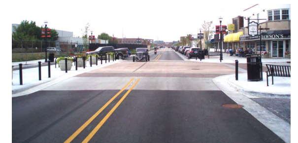
Raised Intersection with Pavement Change
