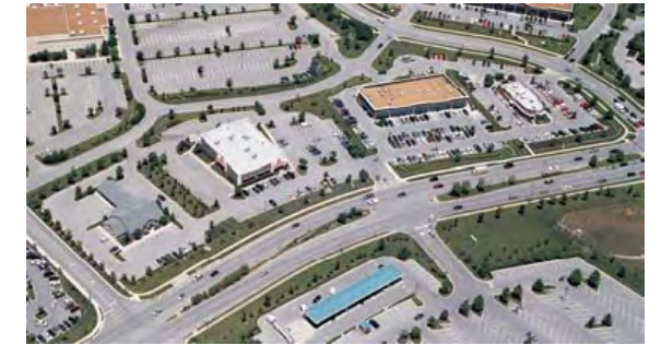
Common access easements are utilized along arterials and internally to minimize points of conflict along streetscape
