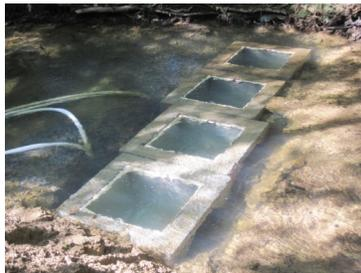
These concrete boxes are part of the stream restoration research project. Shown here, they are approximately 90% installed and will be backfilled shortly for stabilization.
